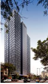
Vinaconex Tower, Hanoi, Vietnam
