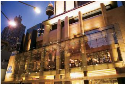
Hilton Hotel Renovation, Sydney
