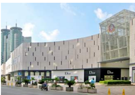
Heyi Road Riverfront Shopping Centre, Ningbo PRC
