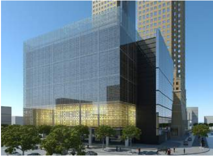
Yuda Palace Hotel and Mall Renovation and Extension, Zhengzhou, PRC
